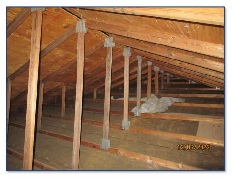
Photograph No. 20: General view of the prefabricated wood roof trusses.
