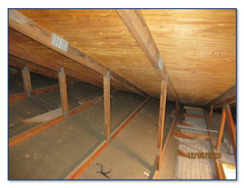
Photograph No. 19: General view of the prefabricated wood roof trusses.
