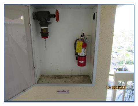
Photograph No. 30: Fire extinguisher & hose valve connector.
