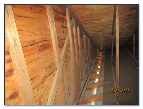
Photograph No. 21: General view of the prefabricated wood roof trusses.
