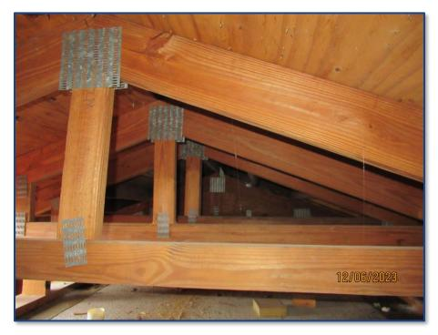
Photograph No. 22: General view of the prefabricated wood roof trusses.
