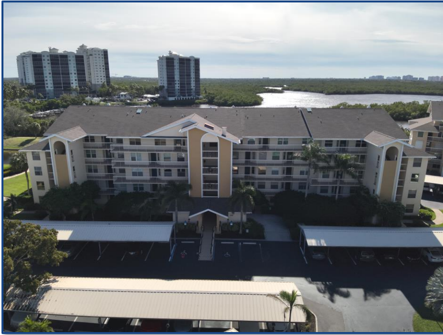
Photograph No. 1: View of the north (front) elevation.
