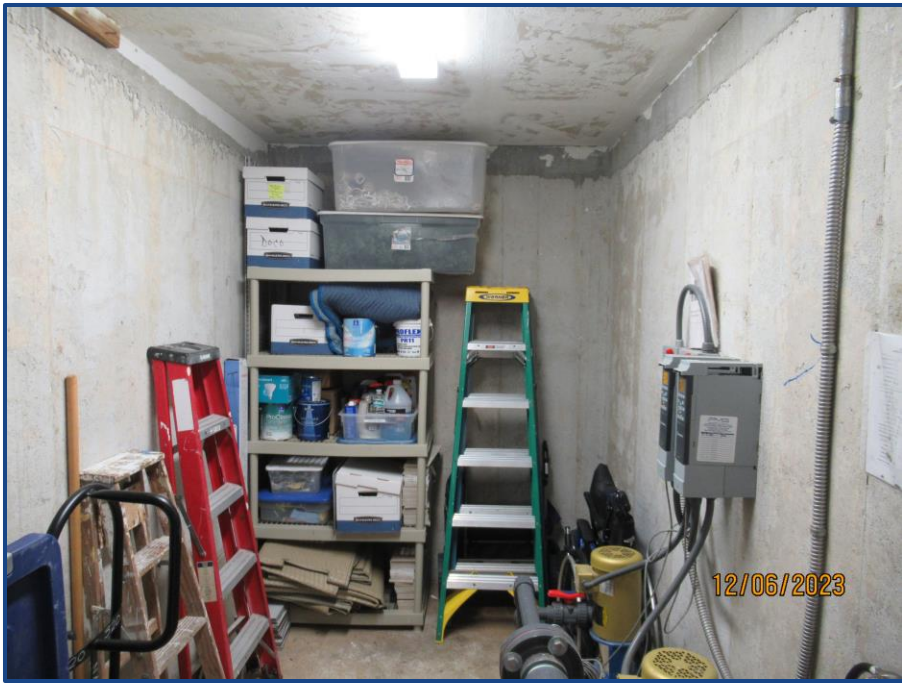
Photograph No. 13: General view of the pump room.
