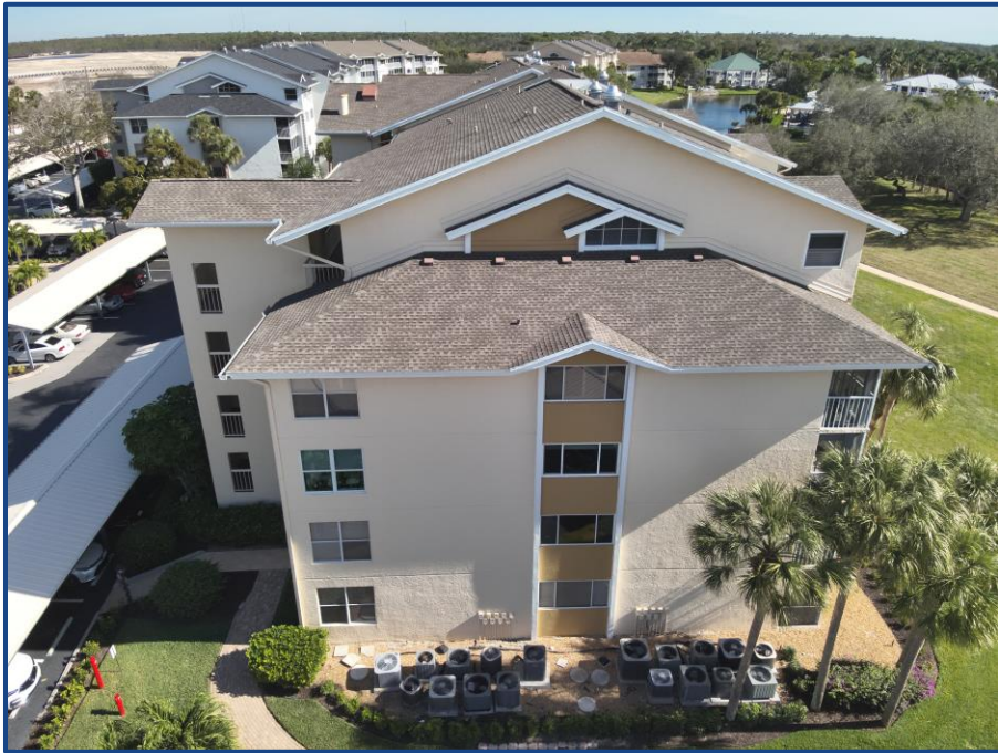
Photograph No. 2: View of the west elevation.
