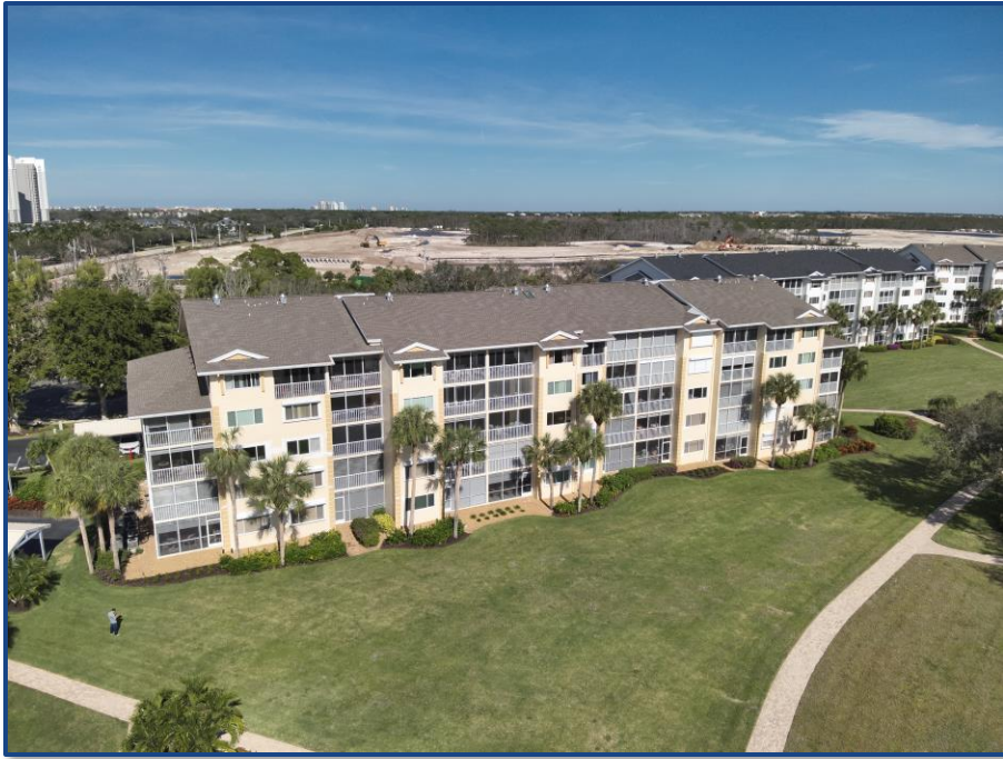
Photograph No. 3: View of the south elevation.
