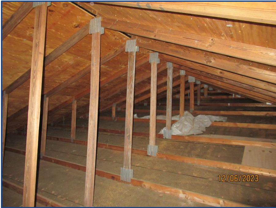
Photograph No. 20: General view of the prefabricated wood roof trusses.
