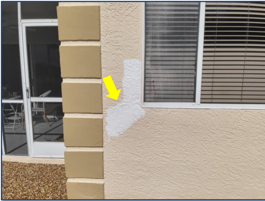
Photograph No. 11: View of previous patch repair.
