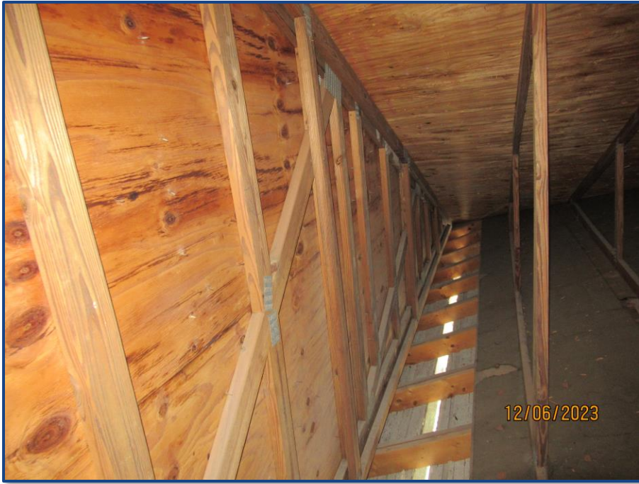
Photograph No. 21: General view of the prefabricated wood roof trusses.
