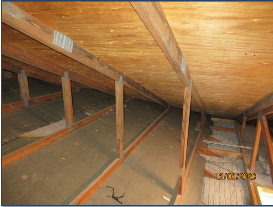
Photograph No. 19: General view of the prefabricated wood roof trusses.
