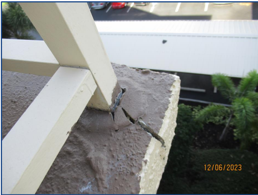
Photograph No. 26: Close-up view of Photograph No. 25.
