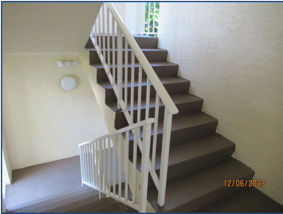
Photograph No. 23: General view of the cast-in-place concrete stairs.
