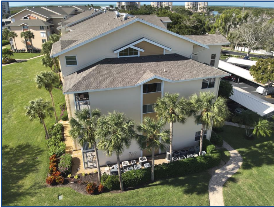
Photograph No. 4: View of the east elevation.
