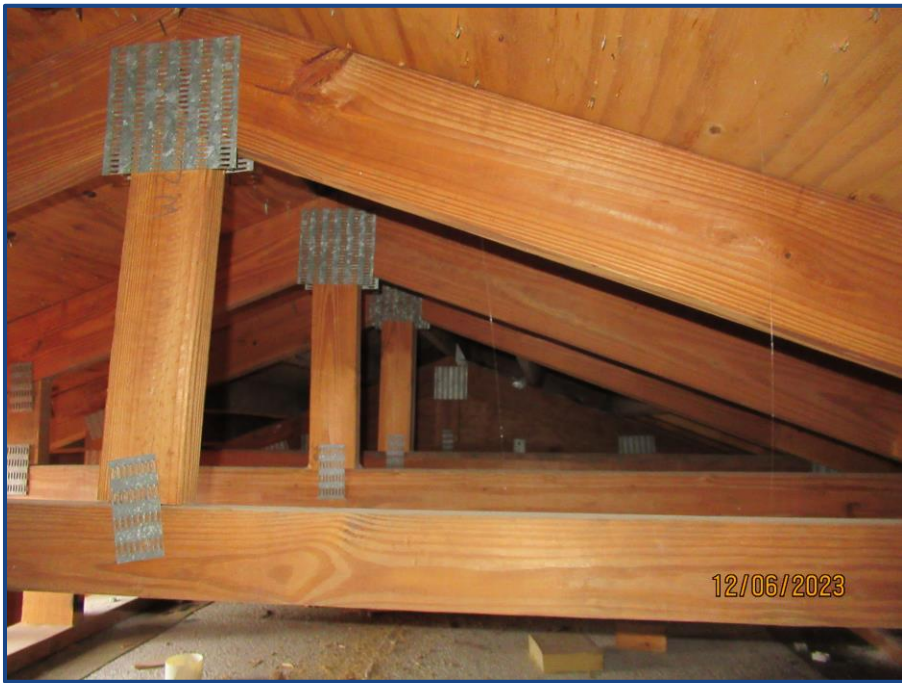
Photograph No. 22: General view of the prefabricated wood roof trusses.
