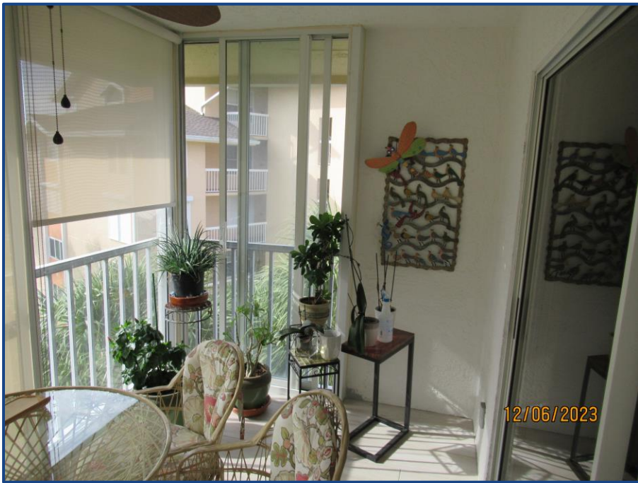
Photograph No. 16: View of the balcony of Unit 408.
